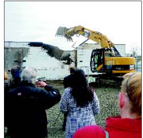
Making way for the new City Hall
